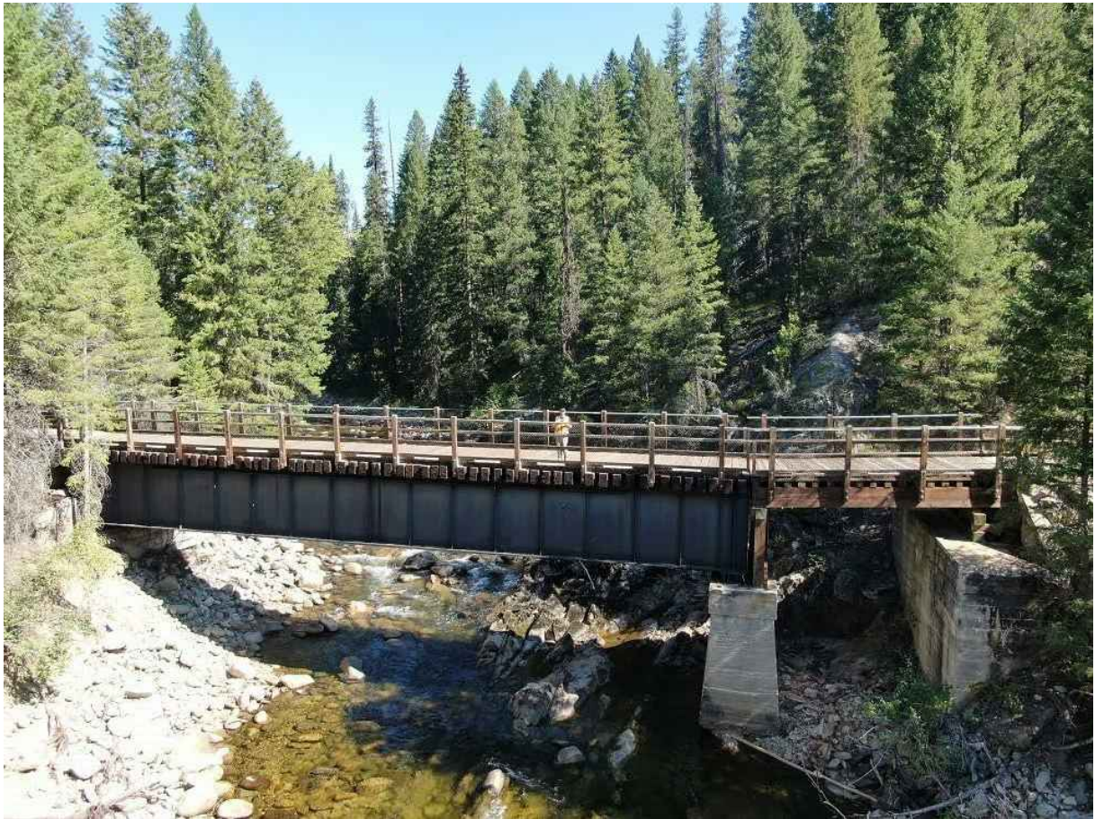
PHOTO 2: OVERVIEW OF BRIDGE LOOKING UPSTREAM
