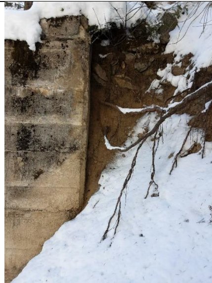
Photo 2. Erosion behind abutment on right bank, upstream side.
