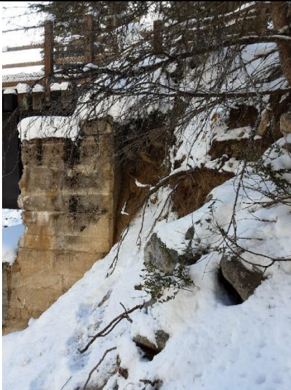
Photo 1. Erosion under abutment on right bank, upstream side.
