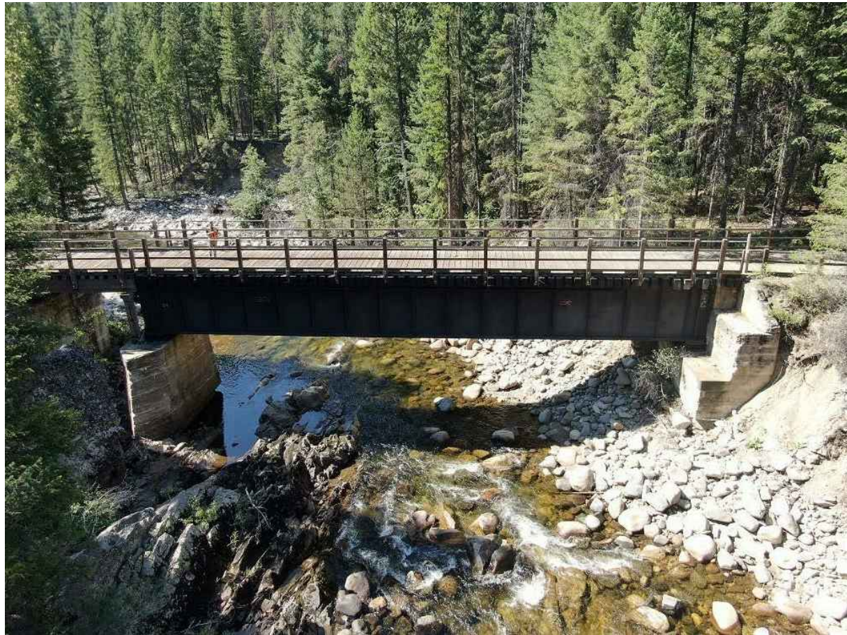
PHOTO 1: OVERVIEW OF BRIDGE LOOKING DOWNSTREAM. REFERENCES TO "RIGHT" AND "LEFT" SIDES OF THE BRIDGE ARE AS SEEN LOOKING DOWNSTREAM
